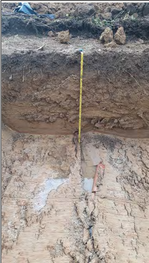
Borehole: TP201 Land drain 0.90m
