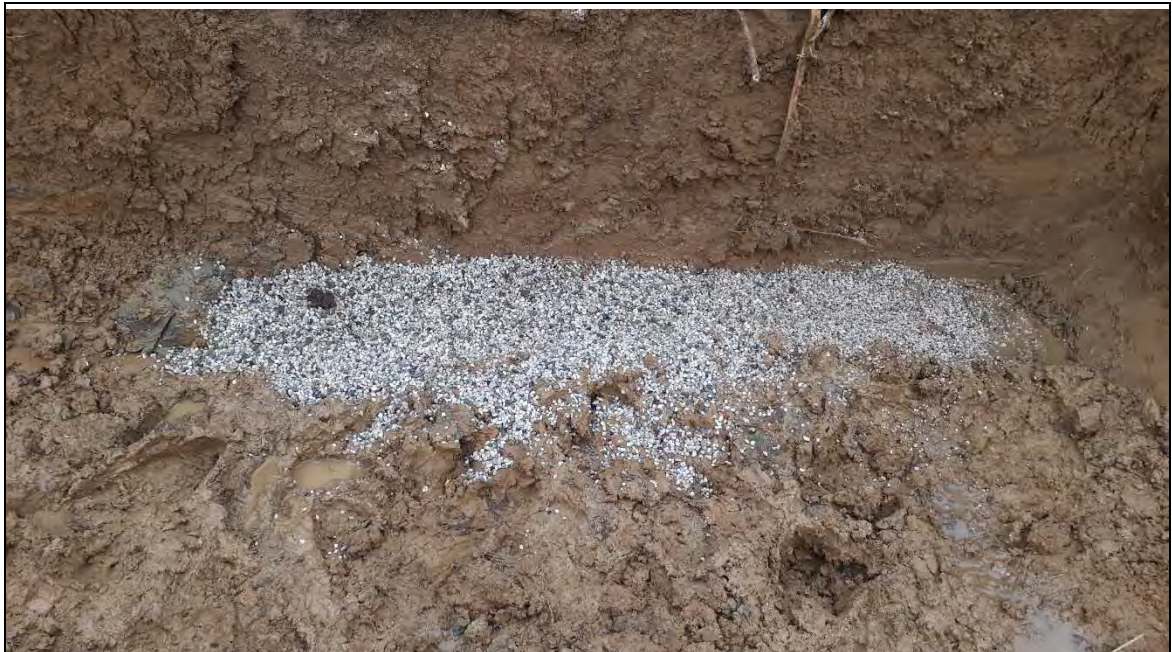
Borehole: TP201 Land drain reinstatement 1.00m
