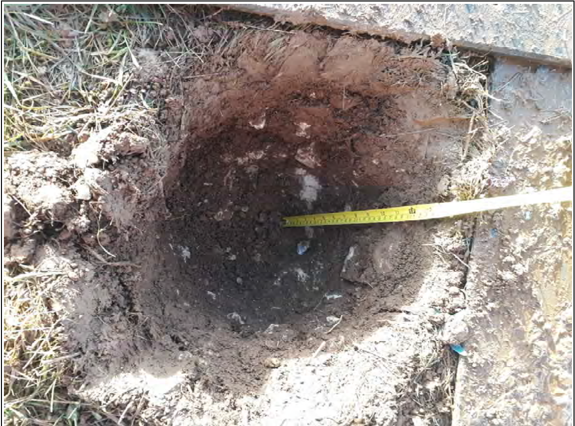
Borehole: DSRCOH308A Pit
